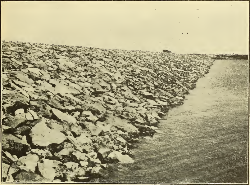
FIG. 33.—Riprapped slope, Minidoka Dam, Snake River, Idaho:
